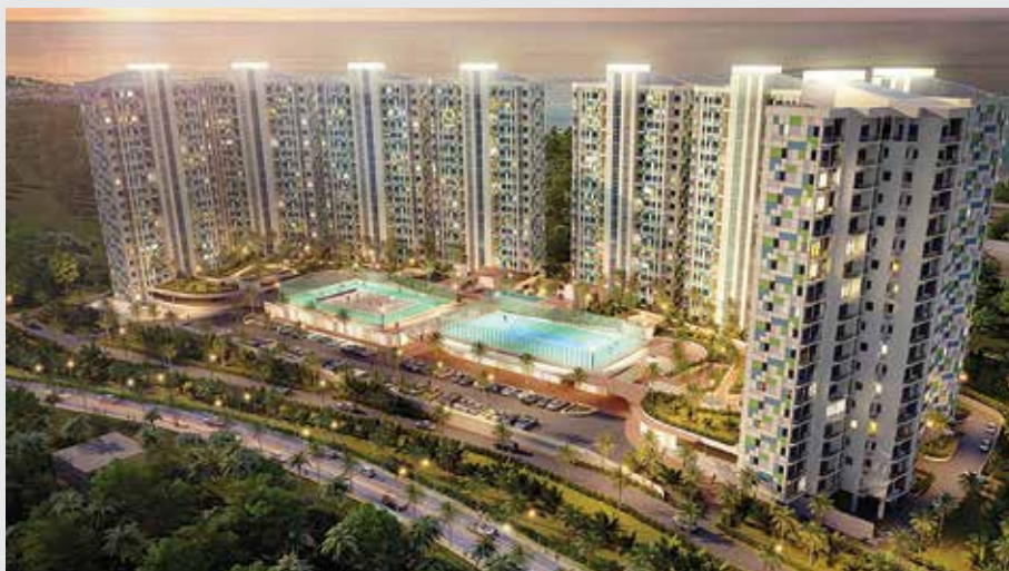
Nhc On-Going Housing Project in Kawe, Dar Es Salaam
